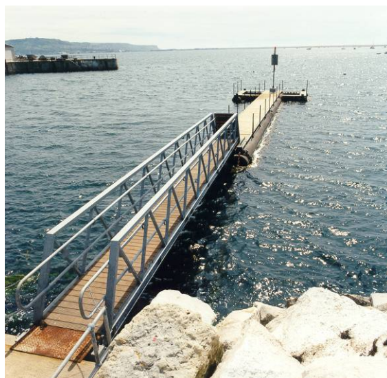
Pontoon raft in Portland Harbour.
